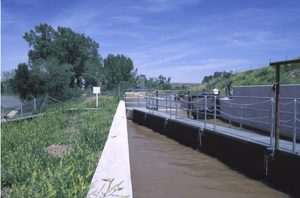
Figure 123.—Louver and walkway. Note river on the left and canal downstream beyond the louver – Example 4 (T&Y Irrigation District).
