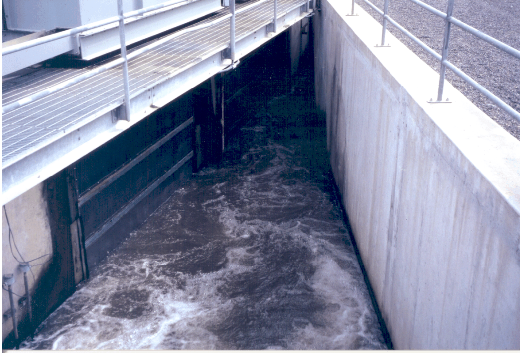
Figure 76.—Traveling screen field site with angled wall – Chandler Canal secondary screen/pumpback structure.
