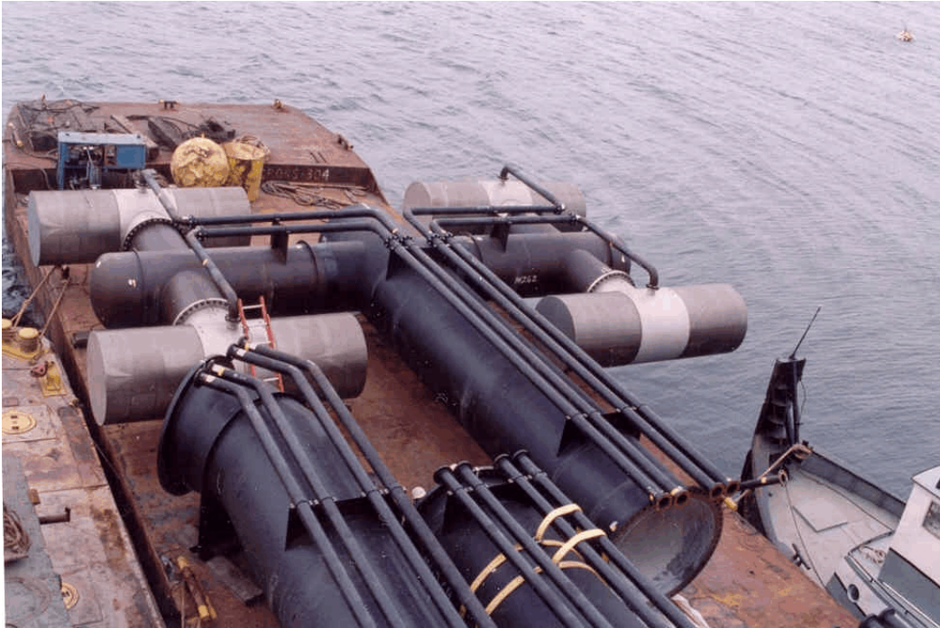
Figure 31.—Cylindrical tee screens on delivery barge for installation at Columbia River Pumping Plant, Oregon.
