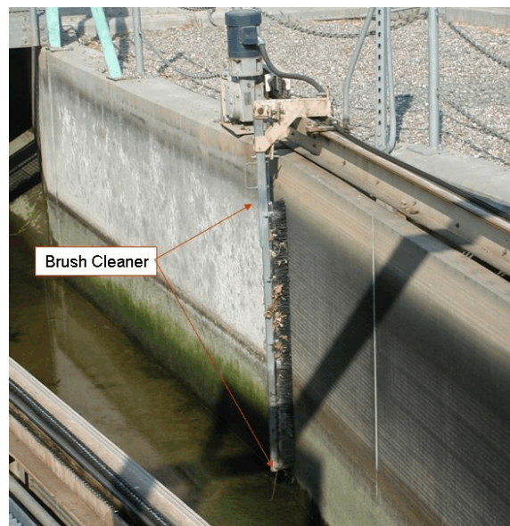
Figure 65.—Mechanical brush cleaner and drive mechanism at Red Bluff Fish Evaluation Facility.
