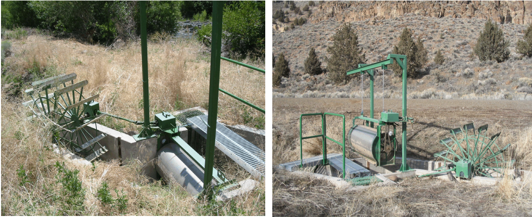
a. Operation – in the dry.
