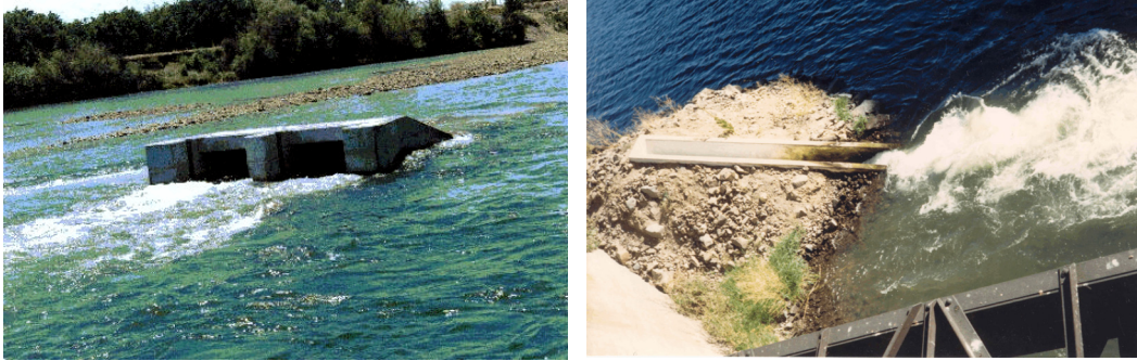
b. Roza Diversion Dam Fish Bypass Right Bank outfall.
