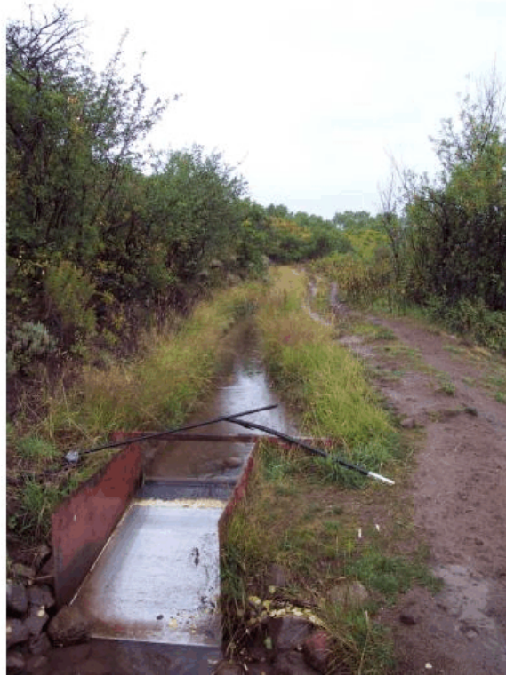
Figure 90.—Coanda screen with low screen slope (Planar) Wildcat Ranch, Carbondale, Colorado.
