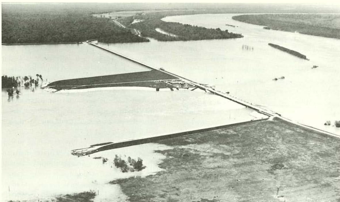
Overbank and Low-Sill Control Structures
