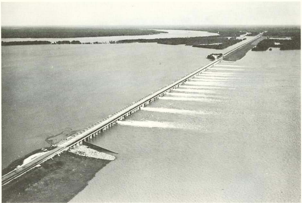
Morganza Control Structure during operation
