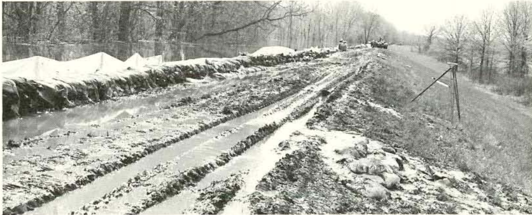
Fabius drainage district, north of pumping station on Fabius levee, looking upstream, 23 April 1973
