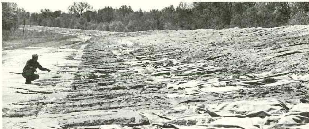
Sny Island drainage district, burlap used to stop erosion caused by seepage on land side of levee upstream from pump station No. 1, looking downstream, 28 April 1973
