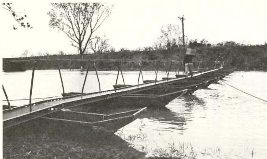
Emergency pontoon foot bridge assembled by Army personnel from Fort Leonard Wood, Missouri
