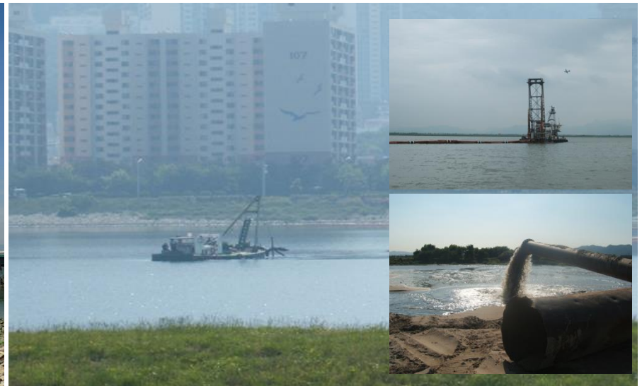
Photos of excavation
