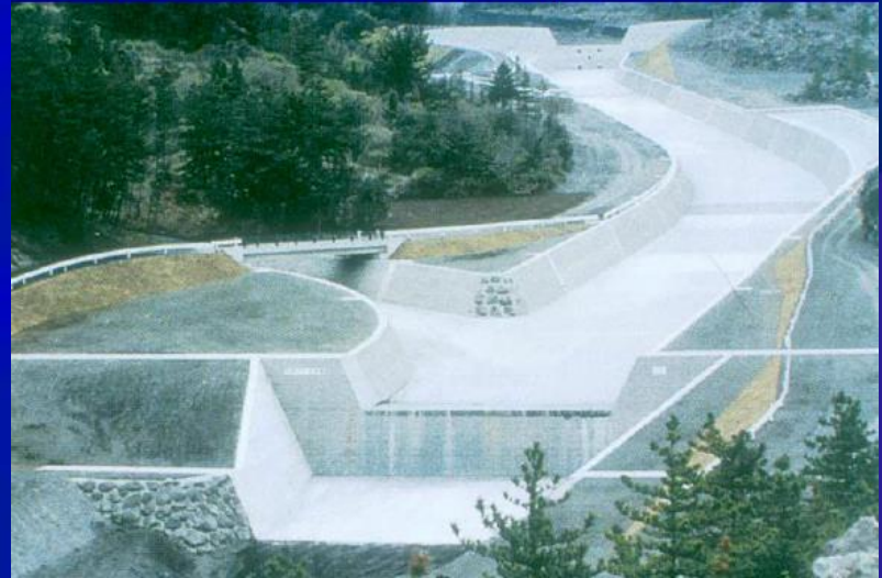
Lined canal with drop structures
