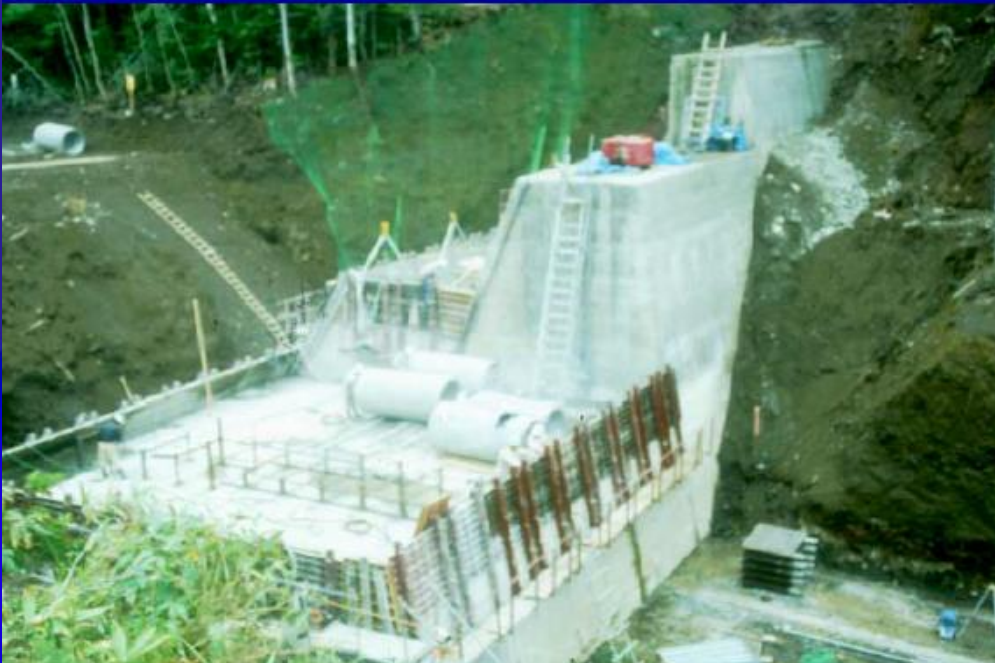
Sabo Dam Construction
