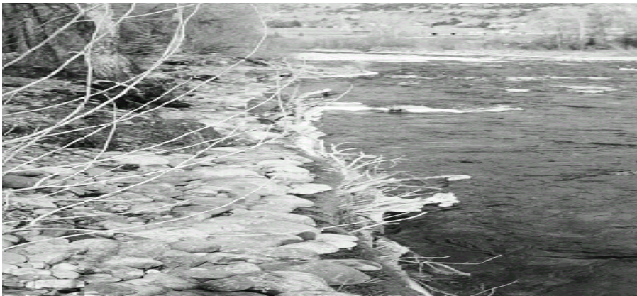
Figure 5.17. Installed log revetment
