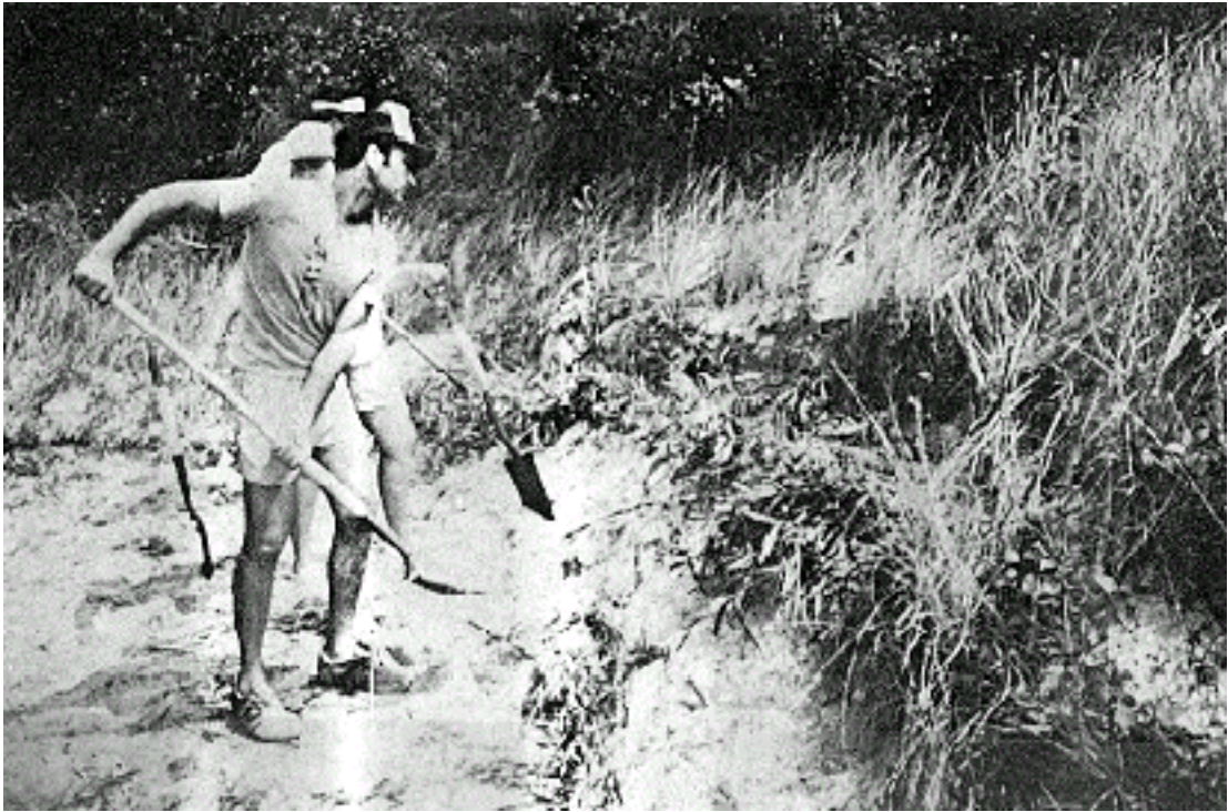
Figure 5.28. Covering brush layers immediately
