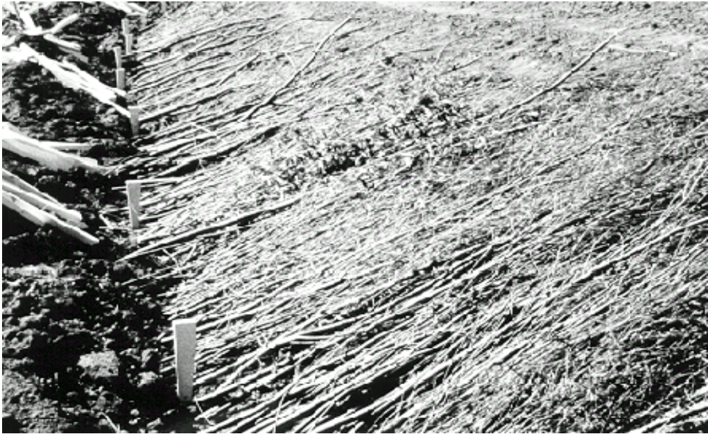
5.26a. Brush placed in a mattress before backfilling
