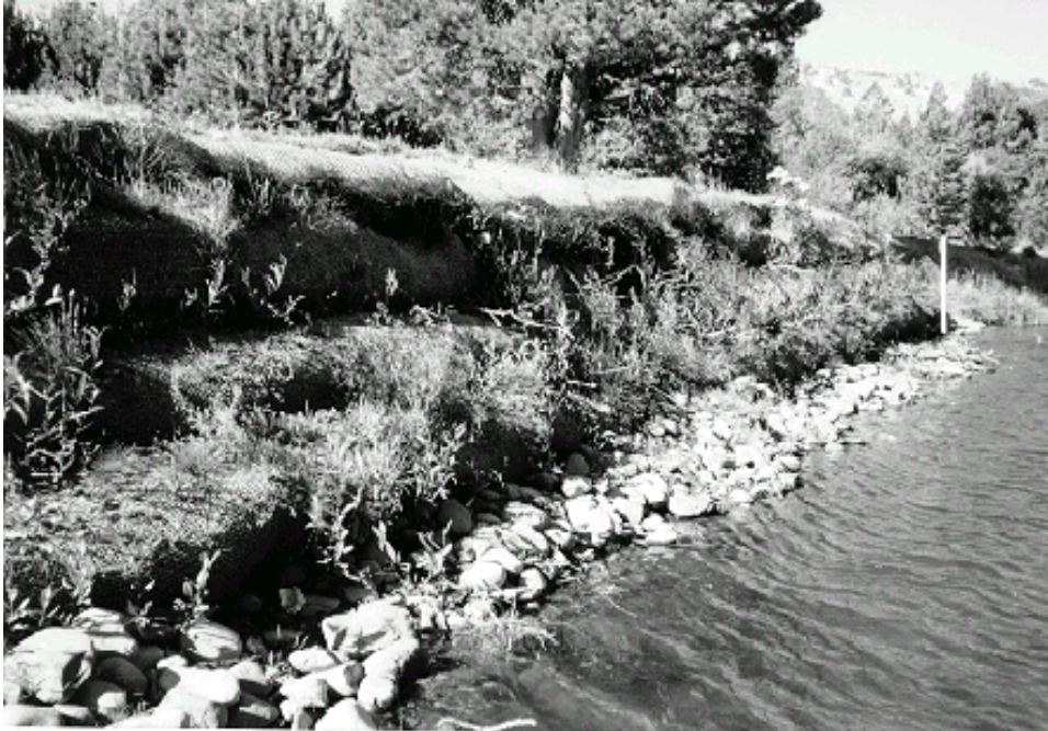
Figure 5.32. Upper Truckee River site after construction
