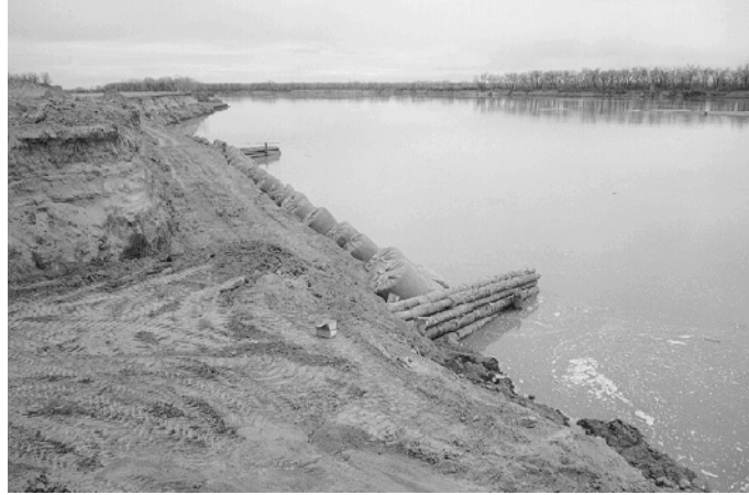
Figure 5.2. Cribs serving as deflection structures
