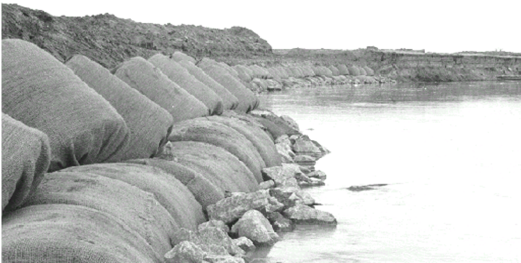
Figure 5.8. Rock toe with hay bale cylinders
