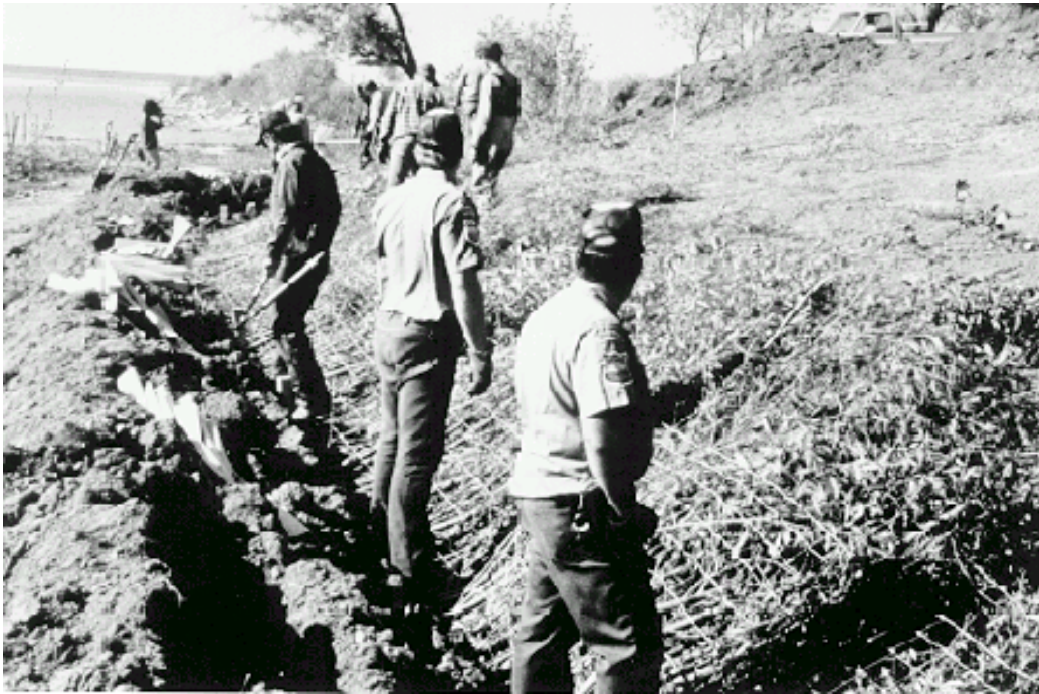
5.26b. Securing woven wire over a brushmattress
