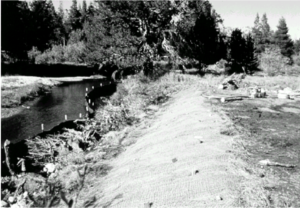
Figure 5.37. Sedges and grasses combination with burlap and woven fabric
