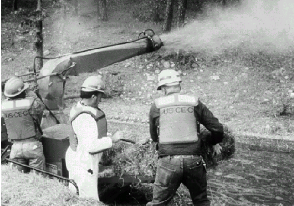
Figure 5.41. Use of hydroseeding and hydromulching equipment
