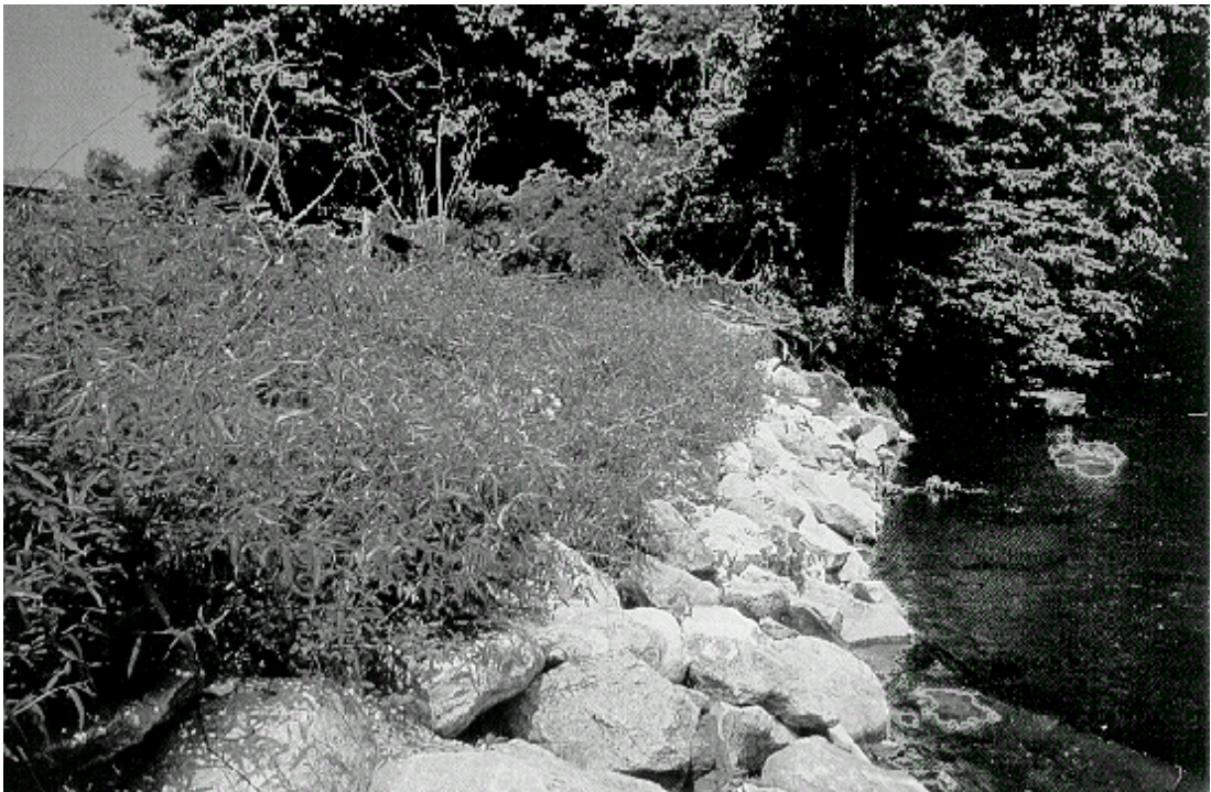
Figure 5.29. Brush layering or branch packing completed (Bowers 1992)
