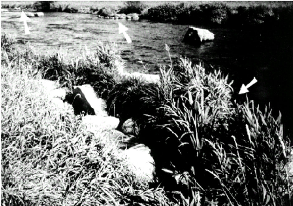
Figure 5.21. Several coir rolls installed (photo courtesy of Bestmann GmbH, Wedel, Germany)
