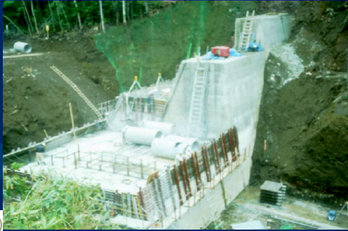
Sabo Dam Construction
