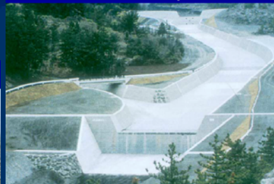
Lined canal with drop structures
