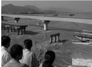
Cuyo bridge failure after Typhoon Maemi (Yonhap)
