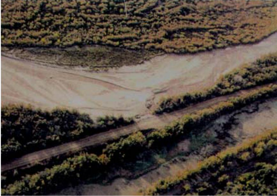
Figure 1.4: Levee breach due to 1991 Tiffany plug (Boroughs, 2005)
