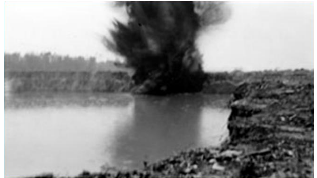
b. Dynamite Blasting Earth Plug
