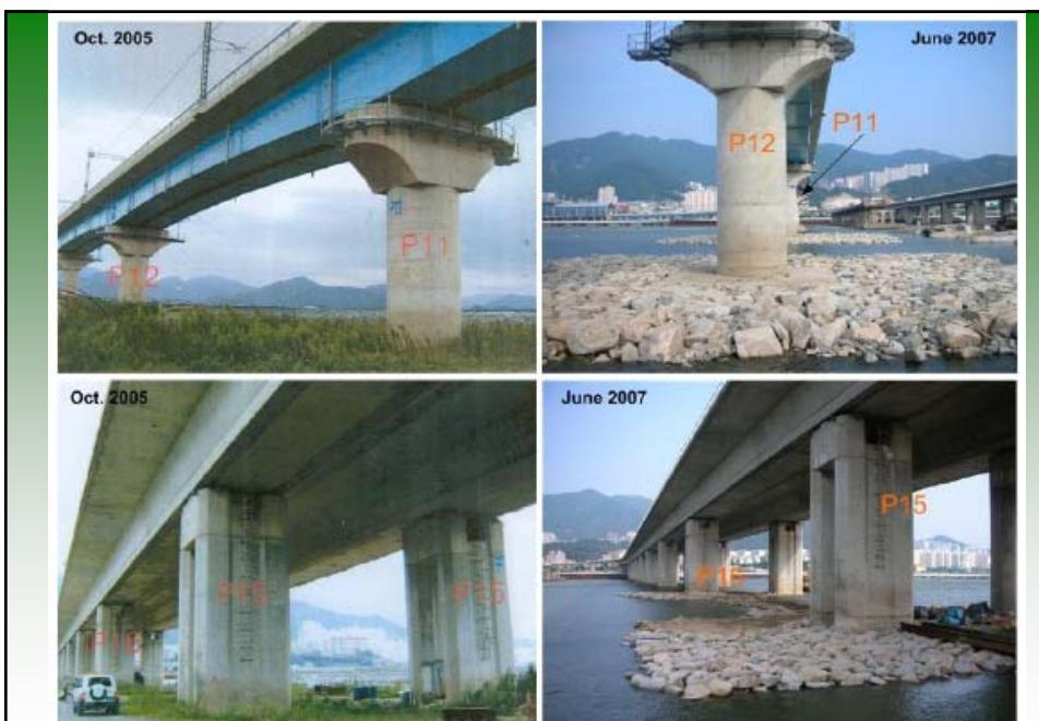
Figure 14. Gupo and Subway Bridge Piers before and after retrofitting construction
