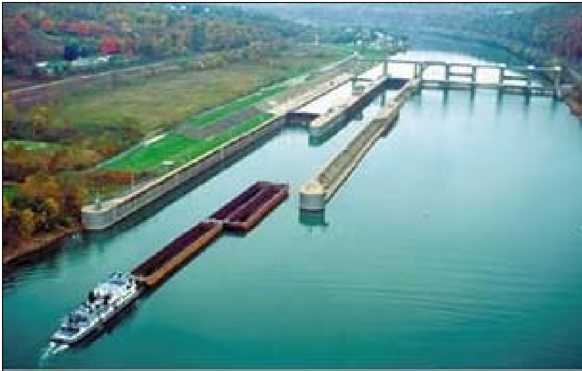
Figure 19: Lock and dam structure in the upper Mississippi River. Sources: U.S. Corps of Engineers
