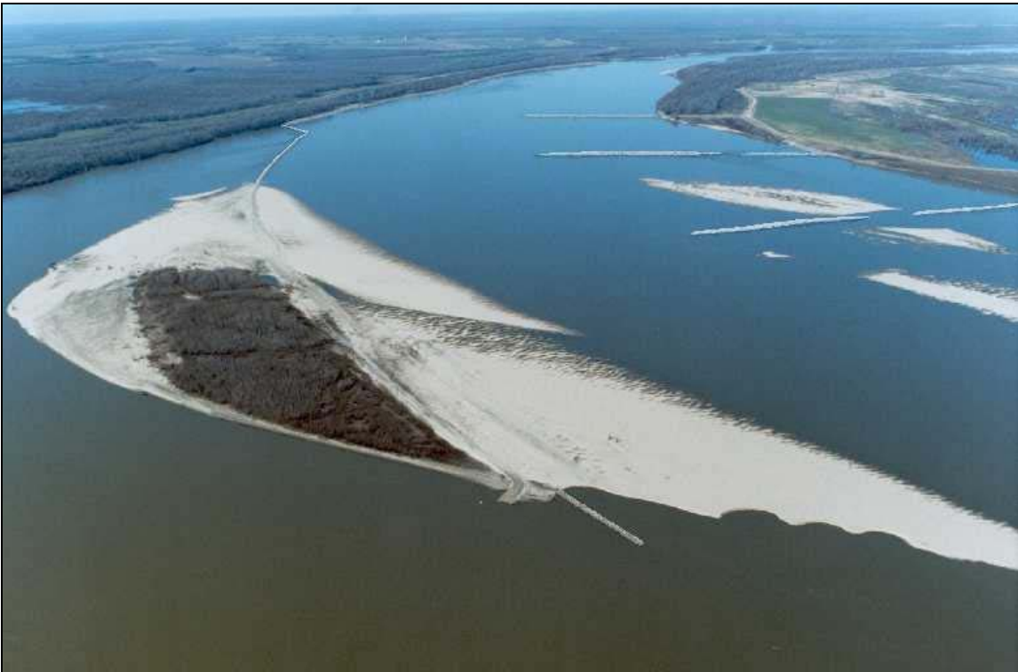
Figure 21: Example of a channel bar formed as a result of revetments Source: U.S. Army Corps of Engineers
