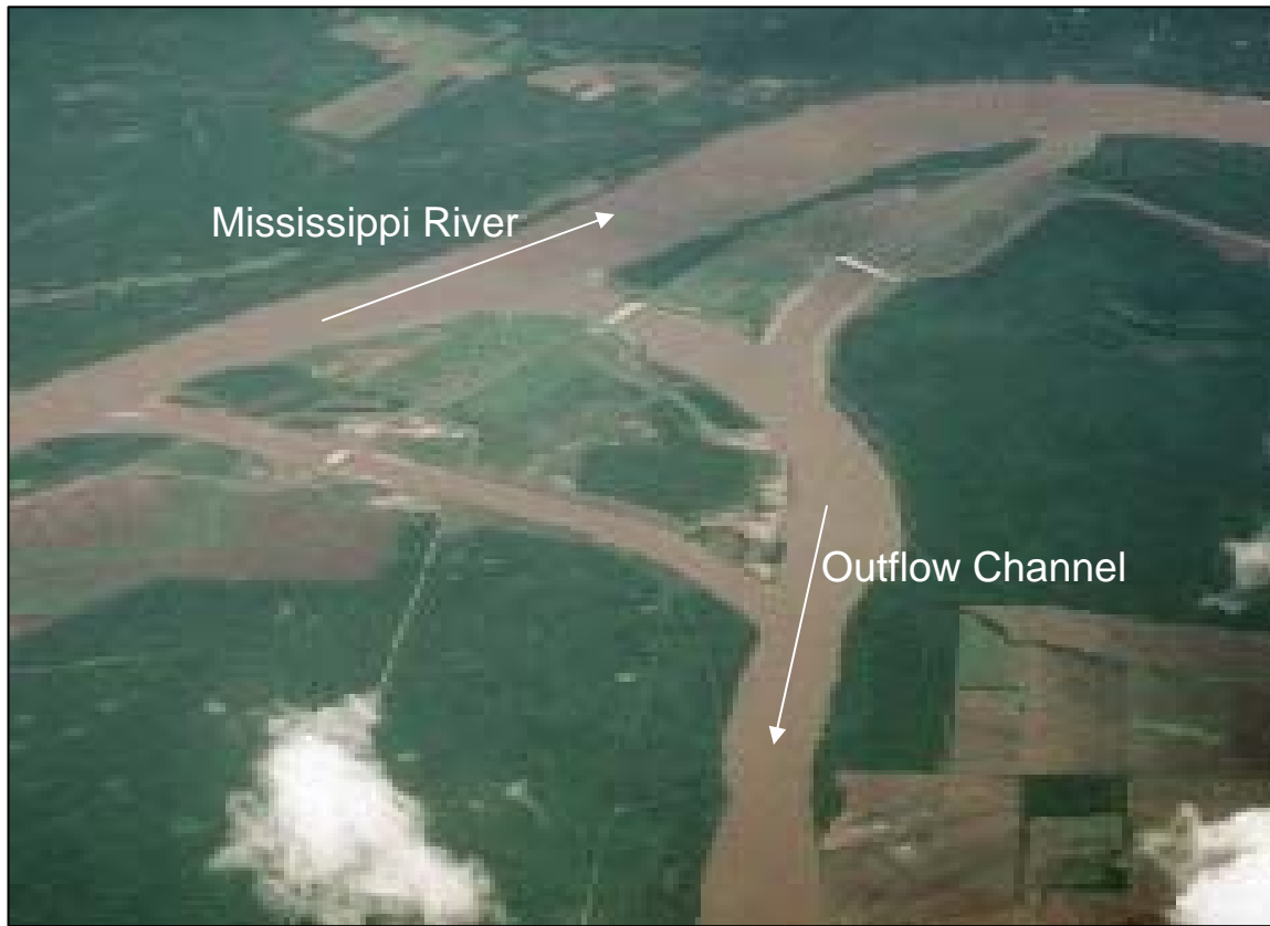
Figure 24: Atchafalaya control structure in the lower Mississippi River. Source: U.S. Geological Survey
