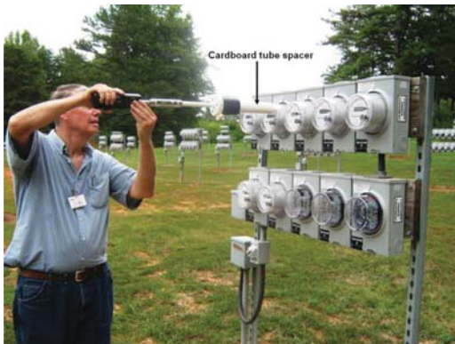
Figure 3. The broadband field probe with an attached cardboard spacer near a rack of 10 smart meters.
