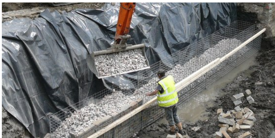
Figure 2-6 Gabions being filled (Gabion1 2016)
