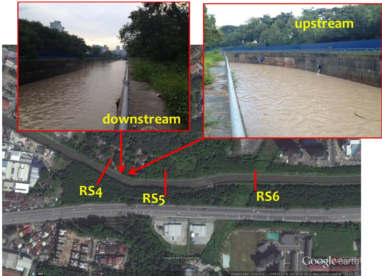
Figure 3 - 11 Site visit photos looking upstream and downstream between River Stations 4 and 5
