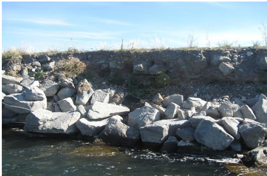
Figure 17 - View of discontinuous rock at mid-bank level (Boyd, 2010)
