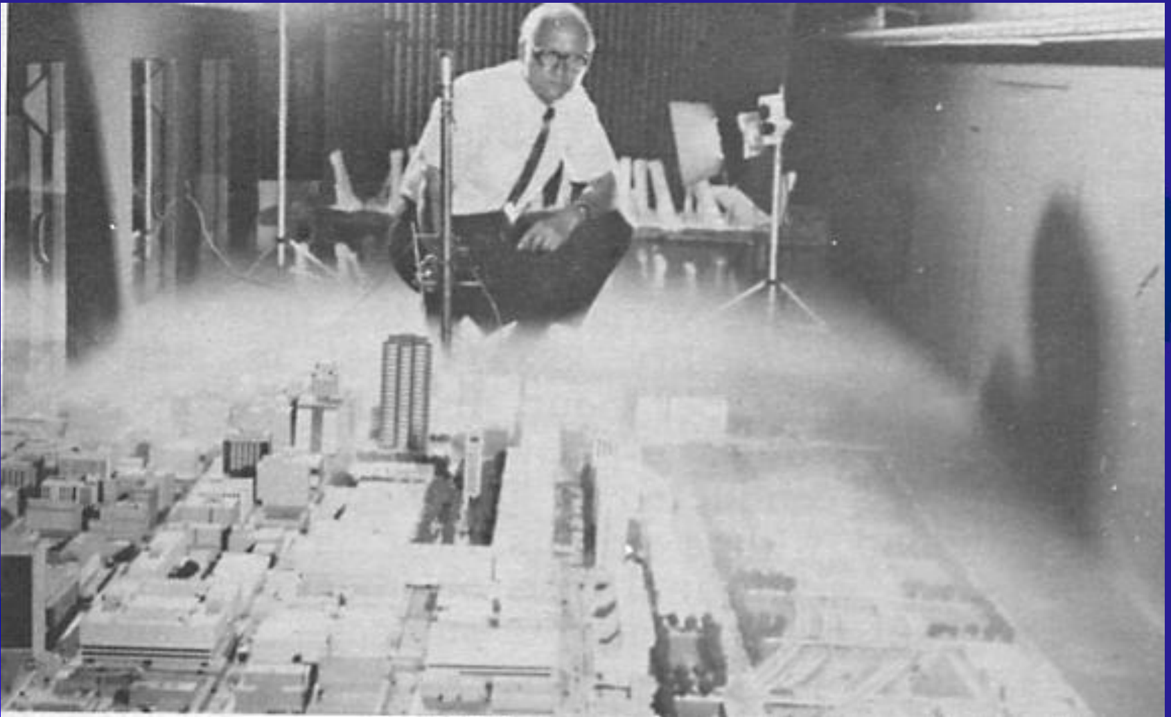
1960's - J. Cermak and the meteorological wind tunnel
