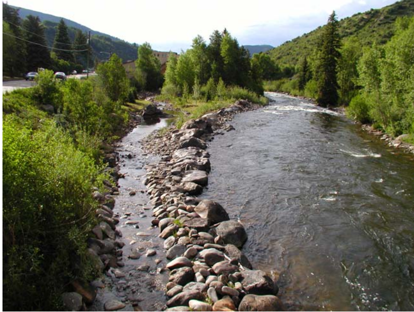
Figure 4.106: Minturn restoration showing the reduction in channel width.
