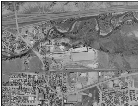
(Above: Aerial view of Eagle River at Gypsum, 1998. Note encroachment of I-70 on meanders near top-center and right corner of photo.)
