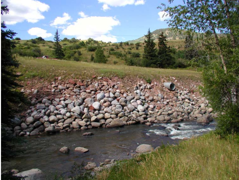
Figure 4.108: Riprap and drainage outfall along Highway 24 downstream of Minturn.
