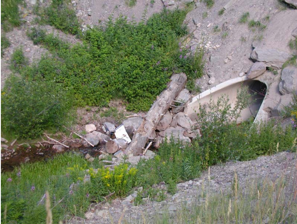
Figure 4.142: Downstream culvert on Squaw Creek.
