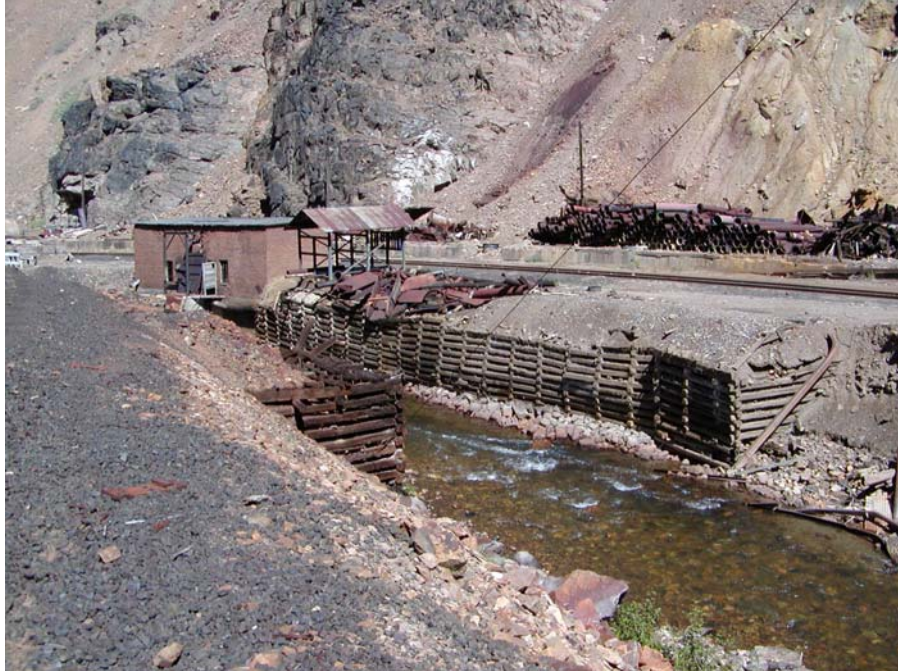
Figure 4.105: Retaining walls along the banks of the Eagle River through Belden.
