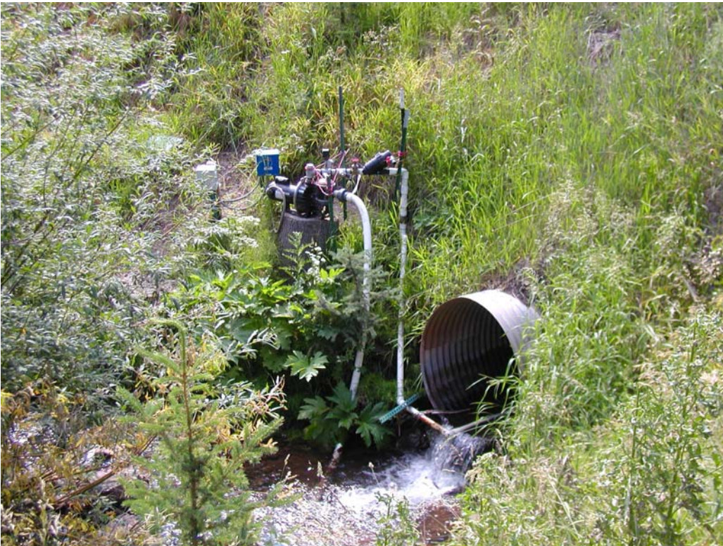
Figure 4.143: Middle culvert on Squaw Creek.
