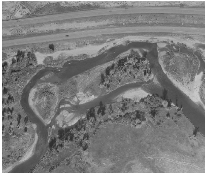
Figure 4.131: Large chute cutoff at Gypsum Ponds SWA.
