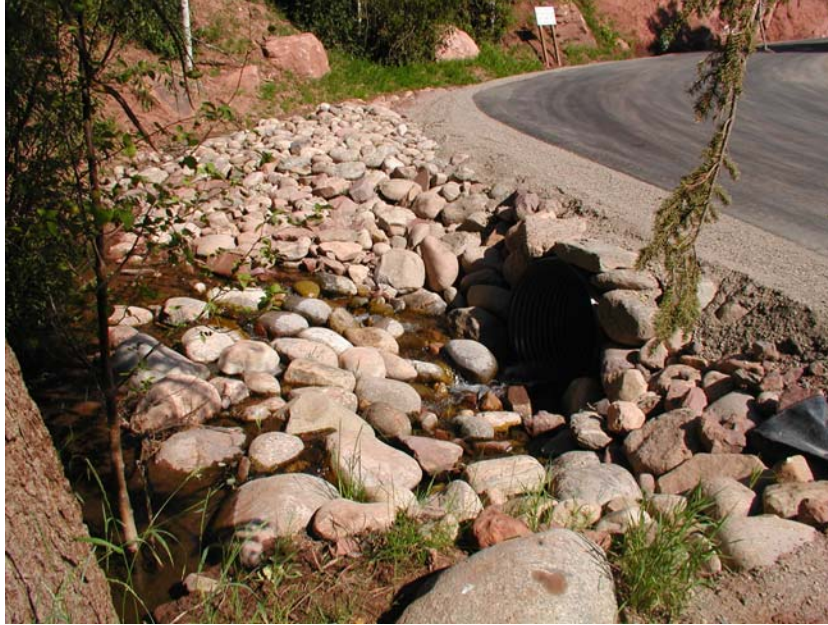
Figure 4.144: Upstream culvert on Squaw Creek.
