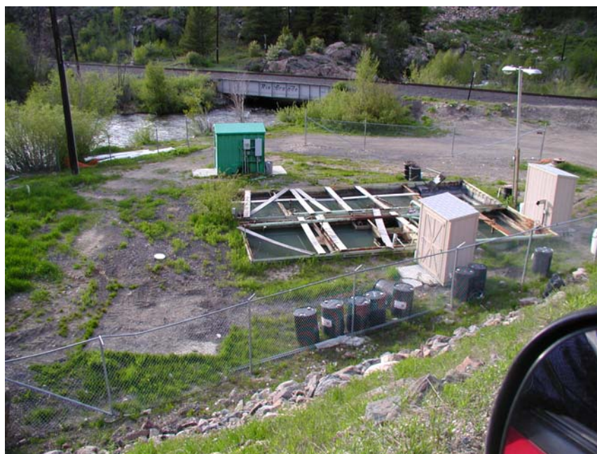
Figure 4.100: Wastewater treatment facility at Red Cliff.
