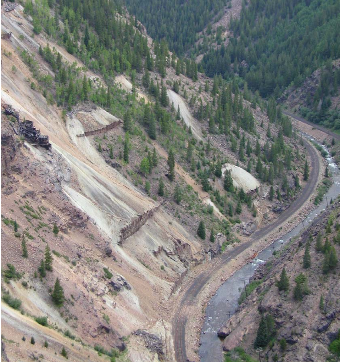
Figure 4.94: Waste rock piles supported by decaying cribs in the Belden area, upstream of the Superfund site.
