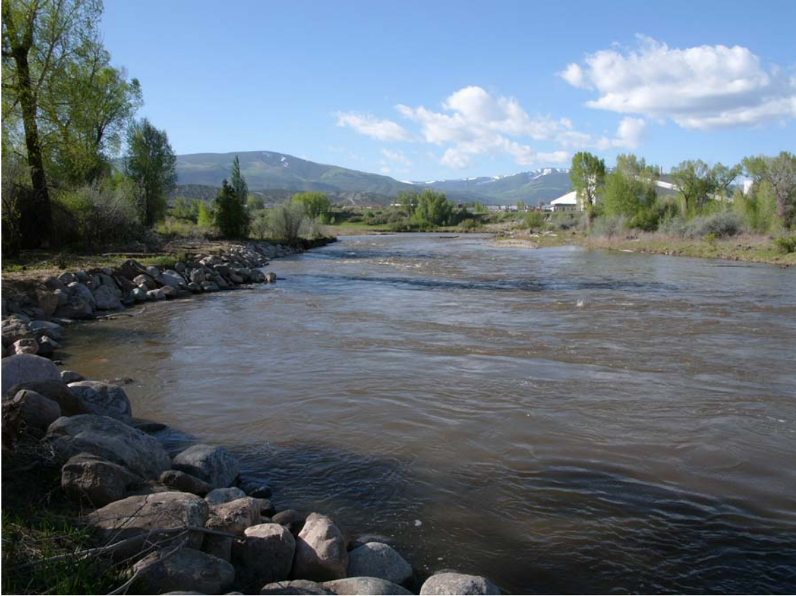
Figure 26: View looking south at Sections 6 and 5 on May 11, 2004. Discharge is approximately 1,600 cfs. Note riprap completed in April of 2004 in foreground.
