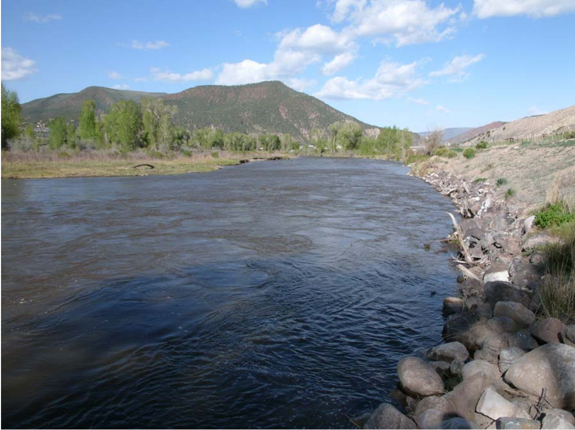
Figure 27: View looking west at Section 7 on May 11, 2004. Discharge is approximately 1,600 cfs. Note riprap completed in April of 2004 in foreground.
