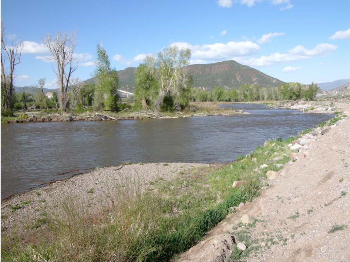
Figure 29: View looking west at Section 2 on May 11, 2004. Discharge is approximately 1,600 cfs. Old log vanes just out of site in foreground and barely visible in background.
